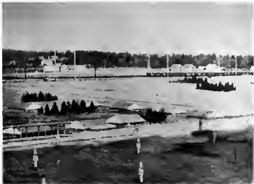
Figure 87. Disruptive pattern painting is used in conjunction with false structures. Houses similar to those in the background are simulated by three dimensional false roofs
